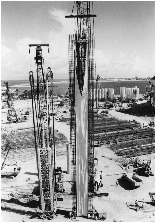
FIG. 2. Hydromill and Reinforcing Cage for Primary Pan
