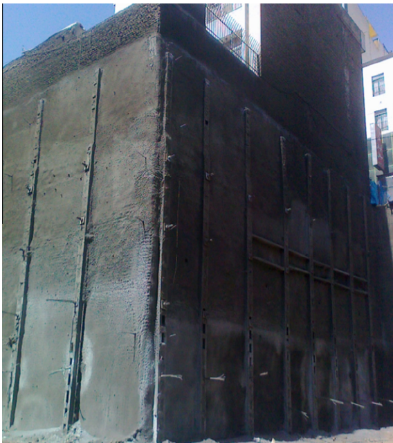
Fig. 4. A schematic view of the 13 m height soil nailing retaining structure on the east side of the project.
