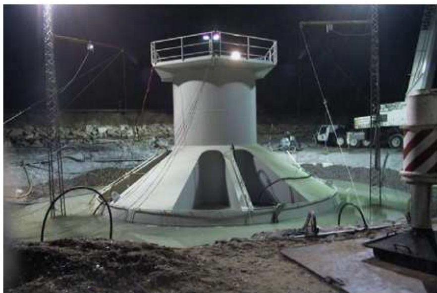
Fig. 1. Bucket foundation after installation in Nov., 2002.
