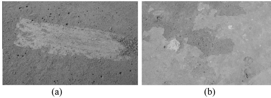
**Fig. 5.** The top surface of filling layer constructed by SSFSCC with improper workability after removing the prefabricated slab seated above. (a) Paste with very porous structure and low strength on the top surface of filling layer, (b) a very thin paste layer with a bubble layer beneath on the top surface of filling layer.
