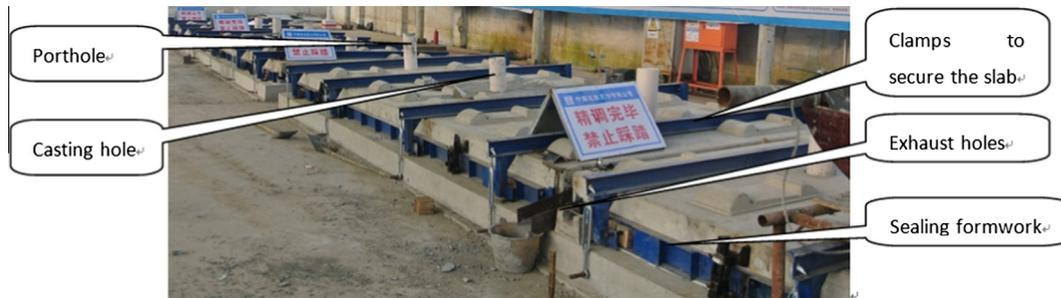
**Fig. 7.** Full-scale field experiment of SSFSCC construction.
