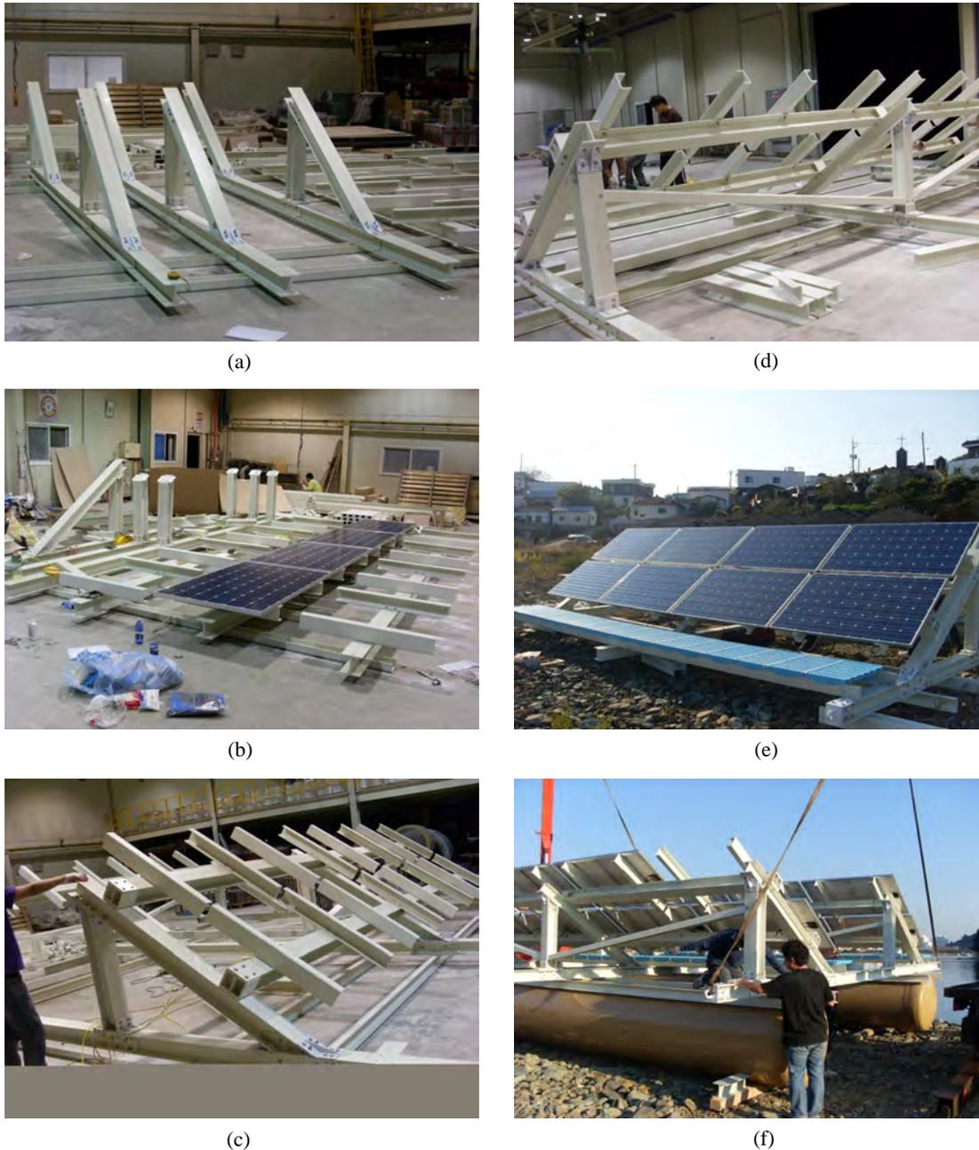
Fig. 15. Fabrication of floating type PV energy generation structure. (a) Fabrication of vertical unit member; (b) fabrication of horizontal unit member; (c) connection between vertical and horizontal unit members; (d) fabrication of vertical bracing and guide; (e) assemble PV panels and (f) attach floating object.
