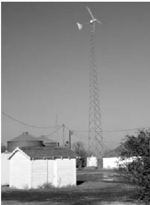
A hybrid system that combines a wind system with a solar and/or diesel generator can provide reliable off-grid power around the clock :
