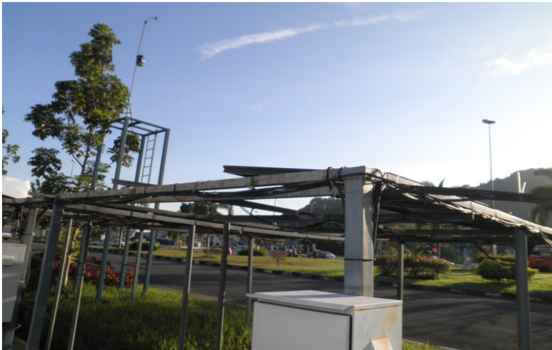
Fig. 1 Weather station and PV array installed in front of CERE, Universiti Malaysia Perlis
