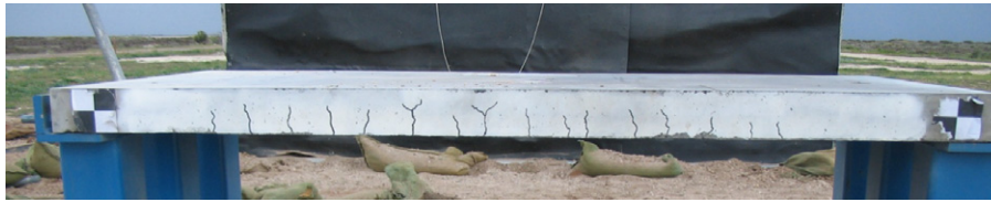
Fig. 13. Cracks in specimen NRC-4.
