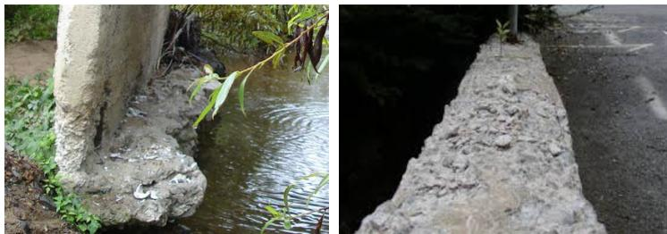
Fig. 1. Concrete degradation caused by frost action.
