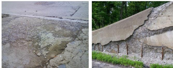
Fig. 4. Concrete degradation caused by crystallization of road defrosting salt.
