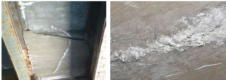
Fig. 6. Leached salts and minerals on concrete surface.
