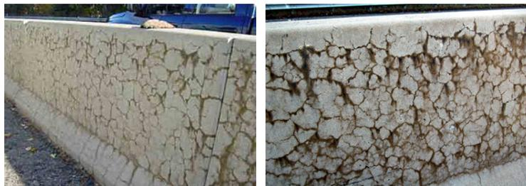
Fig. 3. Degradation by the aggregate expansion paving the way to the further concrete degradation.
