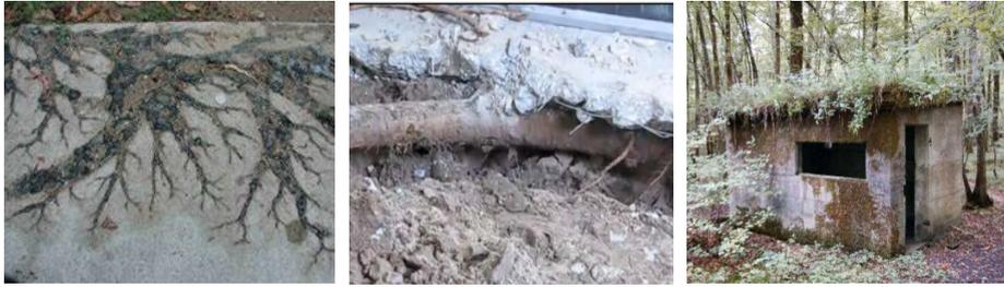
Fig. 2. Degradation of concrete caused by the tree roots and vegetation.
