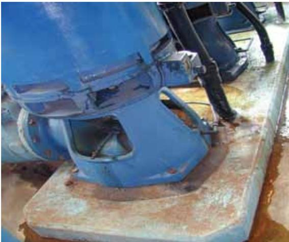
**Figure 10.** Vertical Turbine Pumps – Improper Installation
