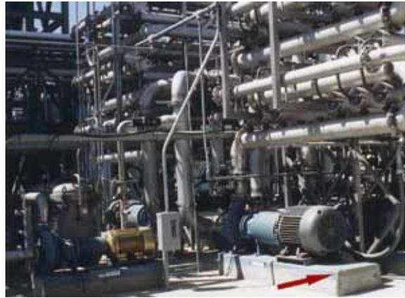
Figure 12. ANSI Pump – Channel Baseplate
