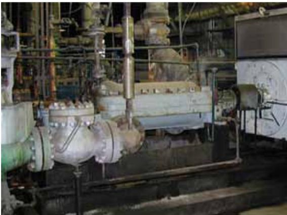
Figure 1. Boiler Feed Pump Unit
