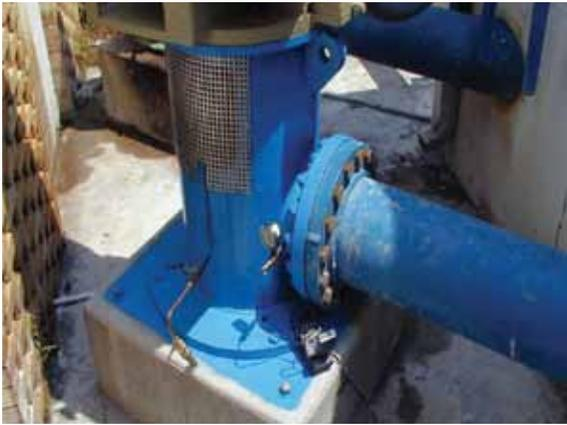
**Figure 9.** Vertical Turbine Pumps – Proper Installation
