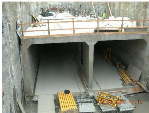
Figure 7 Roof Slab of Side-by-Side Box
