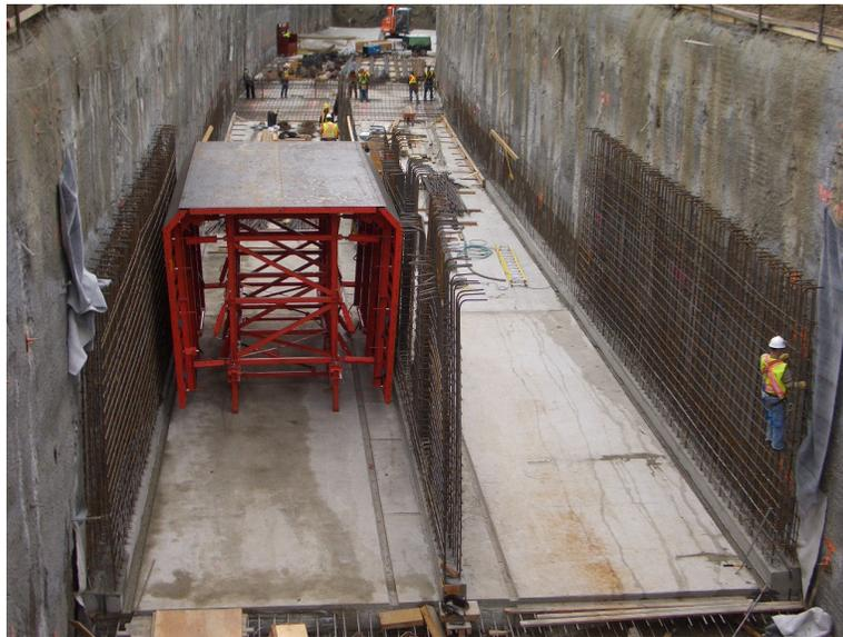
Figure 6 Side-by-side Box Steel Form and Wall Reinforcing
