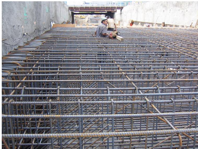
Figure 8 Roof Slab and Wall Reinforcing
