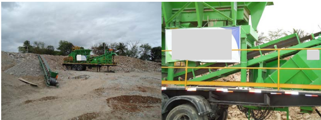
Fig. 4. mobile equipment for removal and crushing.
