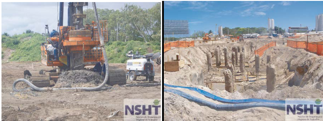
Fig. 2. (a) continuous flight augers; (b) erecting piles.
