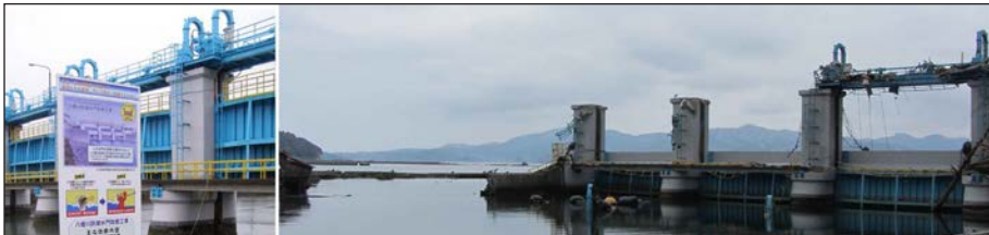
Figure 9. Left: gates on the Hachiman River, Minimisanriku, in April 2010 in the up position (photo courtesy of J. Bourgeois). Right: the same gates in May 2011 after the tsunami. They closed before the tsunami struck, but failure of the sea walls negated their effectiveness (photo: L. Dengler).
