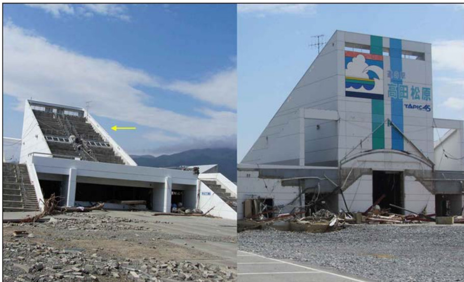
Figure 5. Tsunami evacuation building, Rikuzentakata. Measured water levels were 19 m, shown by the yellow arrow (photos: L. Dengler).
