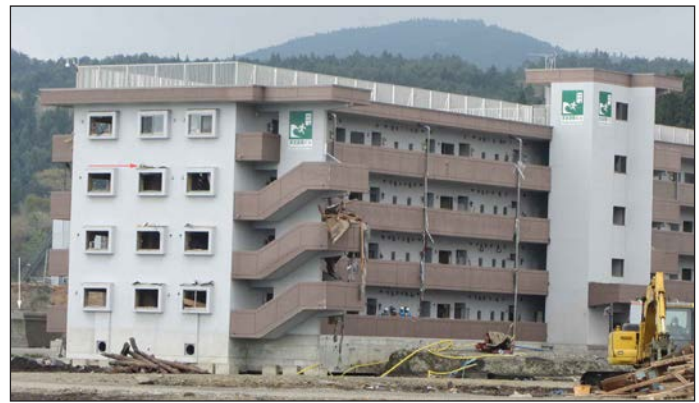
Figure 25. Tsunami evacuation building in Manamisanriku (B on map, Figure 8). The building is adjacent to the sea wall (white arrow on the left). The tsunami left debris on the fourth floor windows (red arrow) (photo: L. Dengler).
