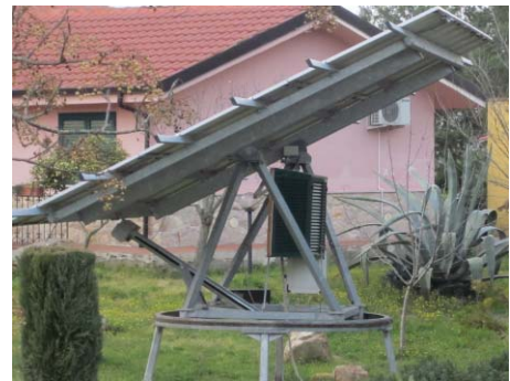
Figure 9. Photovoltaic panel with solar tracking system
