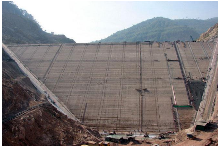
Figure 9: Upstream side of the Nam Ngum 2 dam in Laos PDR
