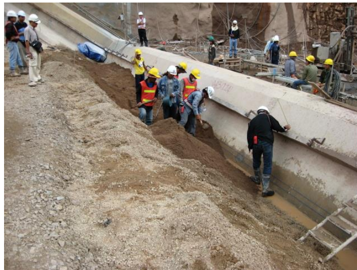
Figure 10: Distributed temperature sensing cable installation at plinth level
