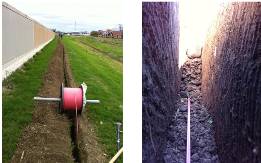
Figure 15: Installation of SMARTprofile sensor in a trench on the protected side of the levee
