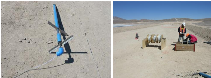
Figure 12: Special packaging for SOFO sensor and cable installation
