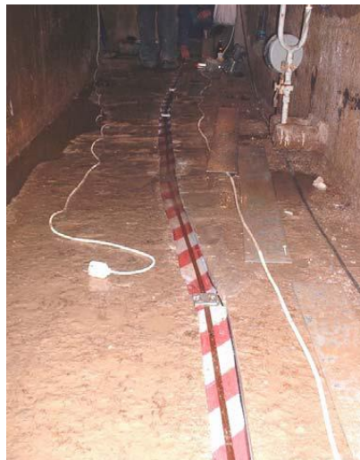
Figure 14: Installation of SmarTape and Temperature Sensing Cable
