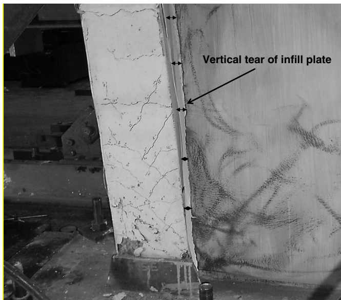
Fig. 5. Base of south column and adjacent infill plate at end of test
