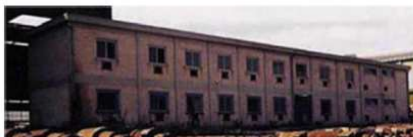
Fig. 1. The building tested within the ILVA-IDEM research project before experimentation.
