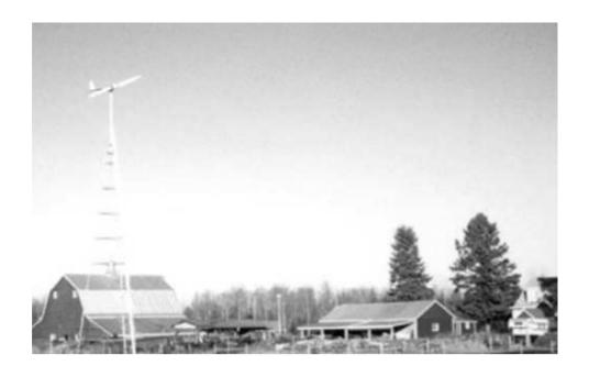
In Clover Valley, Minnesota, this 3-kW Whisper H175 turbine on a 50-foot tower is connected to the utility grid to offset the farm's utility-supplied electricity
