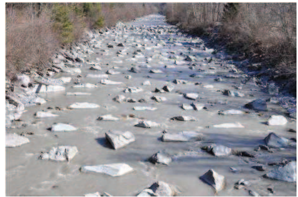
Fig. 3. Upstream view of UBR at the Landquart River, Switzerland, with specific discharge q \approx 0.28 \text{ m}^2/\text{s} (image by authors)
