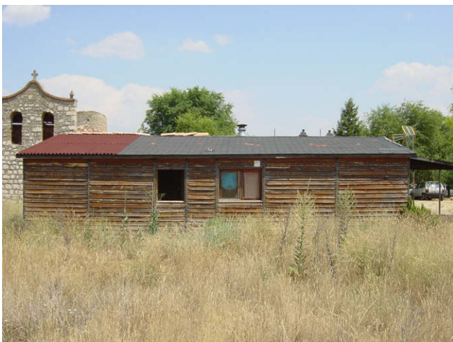
Fig. 6. Western facade of wooden house.
