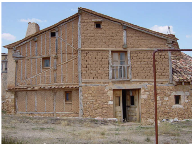
Fig. 4. Southern facade of the adobe house at the present moment.
