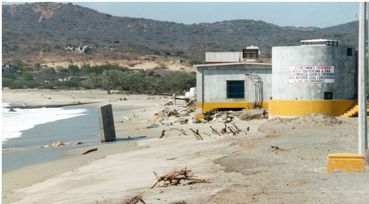
Figure 6 – Desalination Plant Intake Beach Well Erosion
